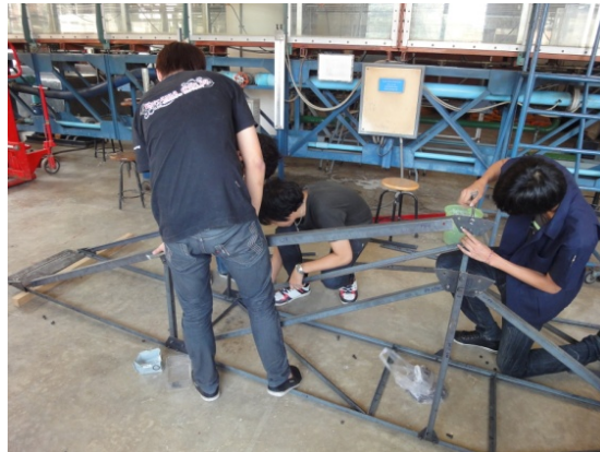
Figure 10: Bridge Structure Joints: TU Bridge Design Team
