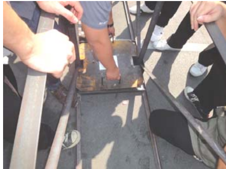
Figure 6: Loading Plate Installation
