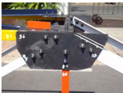
Figure 2: Bridge Structure Joints
