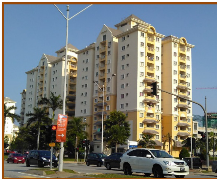
Figure 4: The first case study, colonial architectural style apartment.
