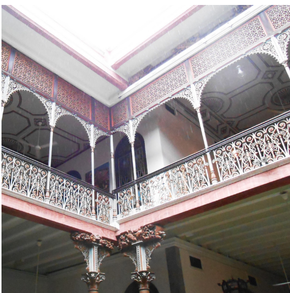
Figure 5: Victorian Scottish cast-iron columns and railings.
