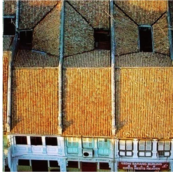
Figure 3: Courtyard enhanced ventilation and interior lighting. (Source: Penang Shophouse, 2017)
