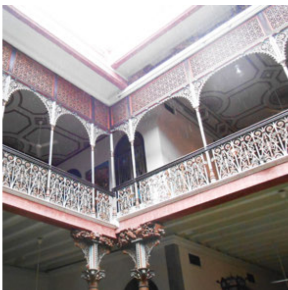
Figure 5: Victorian Scottish cast-iron columns and railings.
