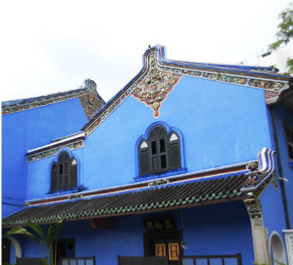
Figure 7: Terracotta roof tiles, decorative mosaic porcelain and painting work on gables & lime plaster and lime wash paint.
