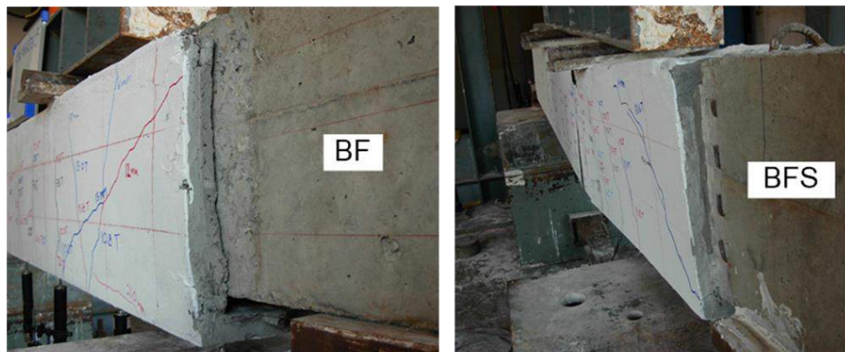
(a) Separation of Ferro-cement from the beam due to the shear flow
