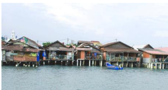
Figure 19: Districts of site that comprises the Clan Jetties.
