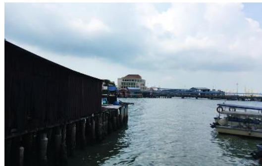
Figure 13: A view from Clan jetty.
