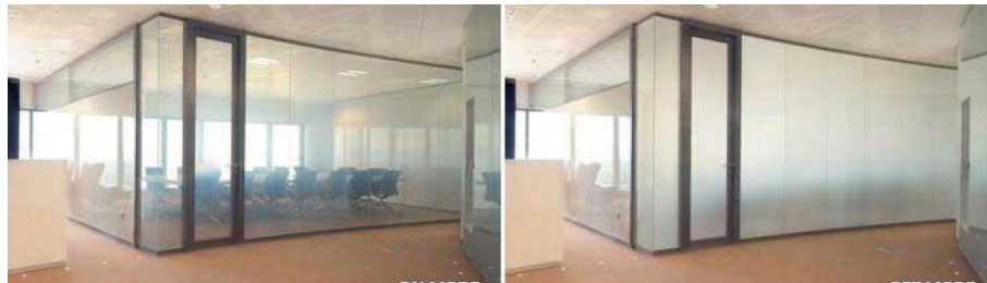
Figure 1. Windows made from photochromic glass
