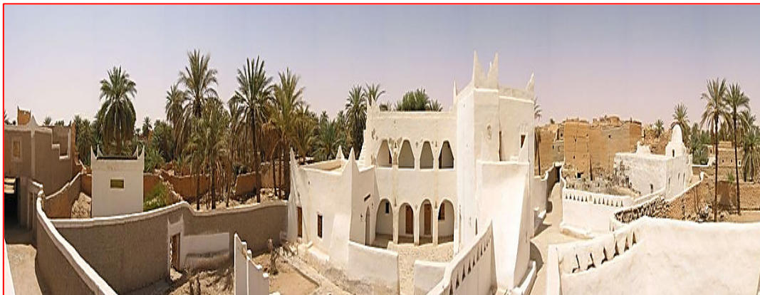
Figure 3: Roof building in Ghadames city
