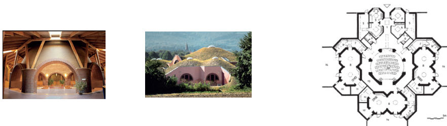
Kindergarten, Sorsum, Germany-Exterior walls, plinth: Porous bricks. Roof: Mud brick domes, timber structure, covered by 15 cm mineral wool, water and rainproof plastic-covered fabric, 15 cm earth, wild grass vegetation. Completion: 1996, Area: 595 m 2 (Minke, 2013, p. 176-177).
