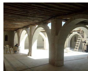
inside of the classrooms
