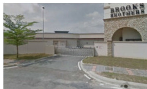
Figure 6: Fencing at Johor Premier Outlet
