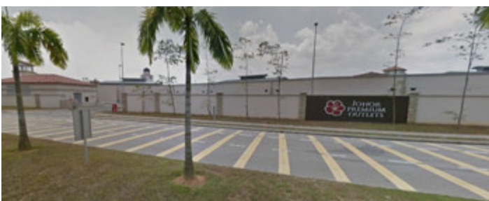
Figure 5: Barrier Wall at Johor Premier Outlet
