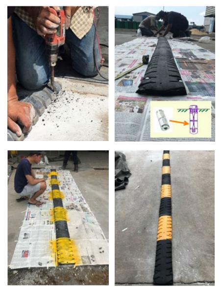
Figure 2: Installation process of bumps built with used pneumatic rubber tires on a local road
