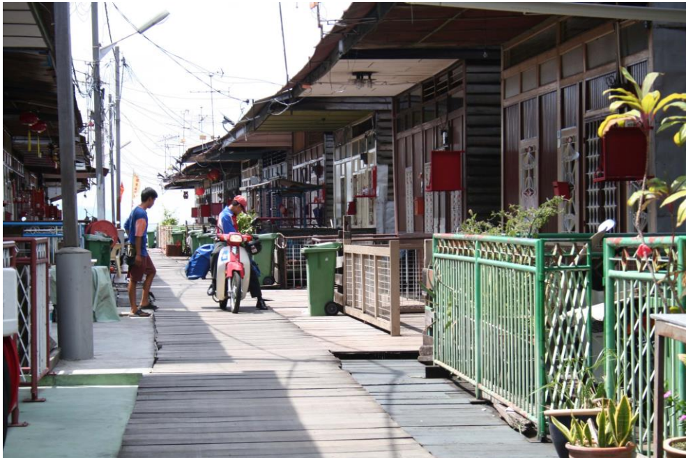
Figure 6: The 2m wide wooden walkway at Chew Jetty-view towards the sea
