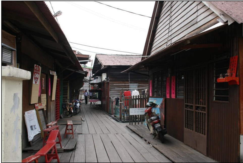
Figure 5: The 2m wide wooden walkway at Chew Jetty-view towards inland
