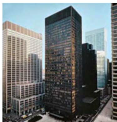
Figure 2. The exterior view of the Seagram Building by Ludwig Mies van der Rohe.
