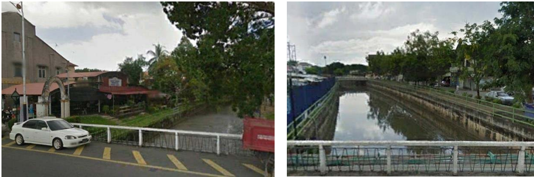
Figure 7: Image of Raja River from Tunku Ibrahim Road, Alor Setar that has become a monsoon drain.
