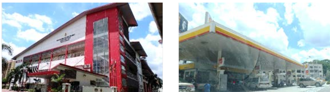
Figure 13: Central MFRD (left), Shell Service Station (right)
