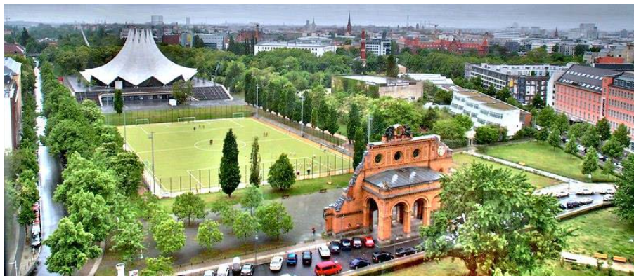
Figure 1: Berlin Anhalter Bahnhof Train Station: Current Status of Façade Fragment (Courtesy of Fonalité/Flickr.com (2013)).
