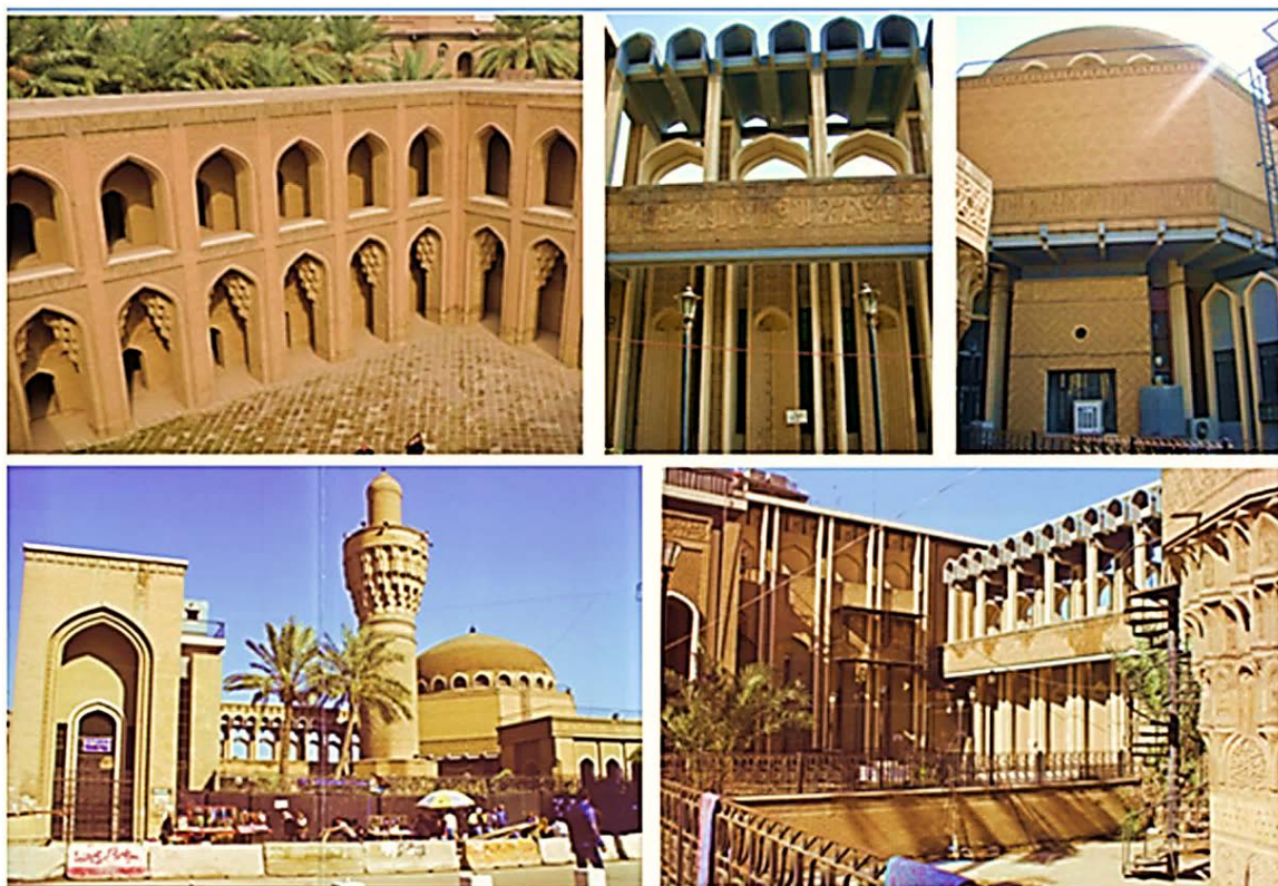
Figure 5: Meaning in the Surface Structure of the Khulafaa Mosque
