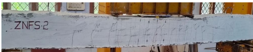
(e) Crack Pattern of ZNFS-2
