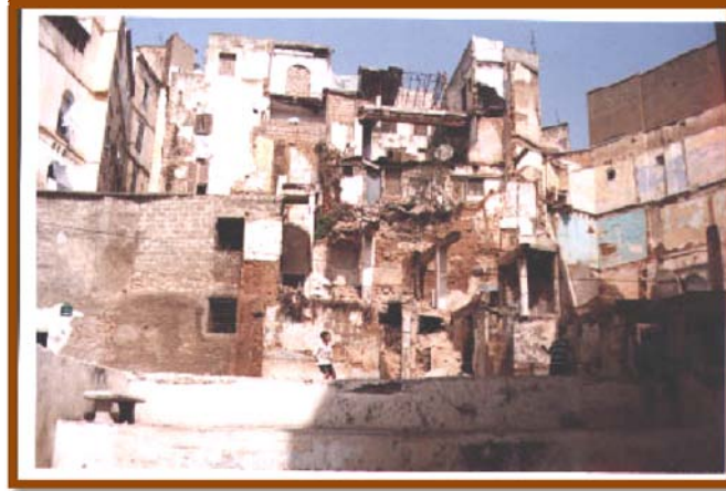
Figure 2: Showing the state of deterioration and dereliction making the Casbah an urban slum in the heart of the capital.
