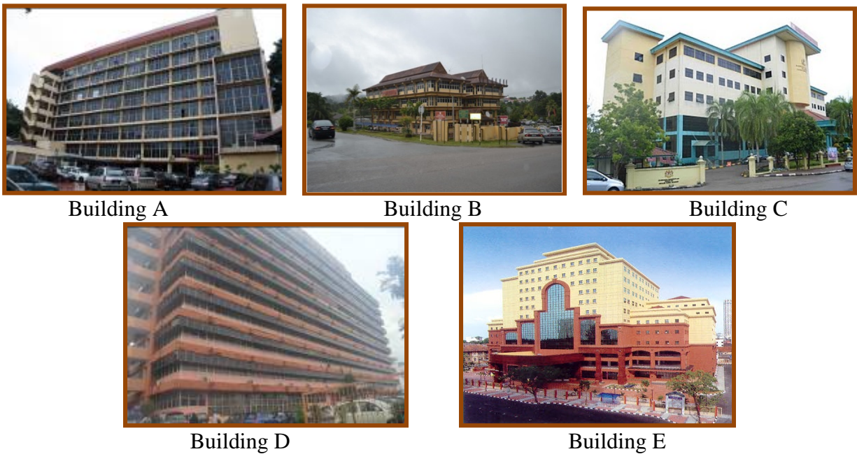
Figure 1: Photos of five government offices : Kuala Lumpur Federal Building(Building A), Gua Musang Federal Building(Building B), Temerloh Federal Building(Building C), Taiping Federal Building(Building D), and Penang Federal Building(Building E).
