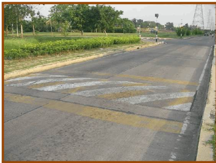
Figure 6: Installed speed hump near crossroad.
