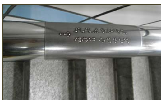
Figure 6: Braille Lettering at Hand Rail (Source: Individual photo collection).
