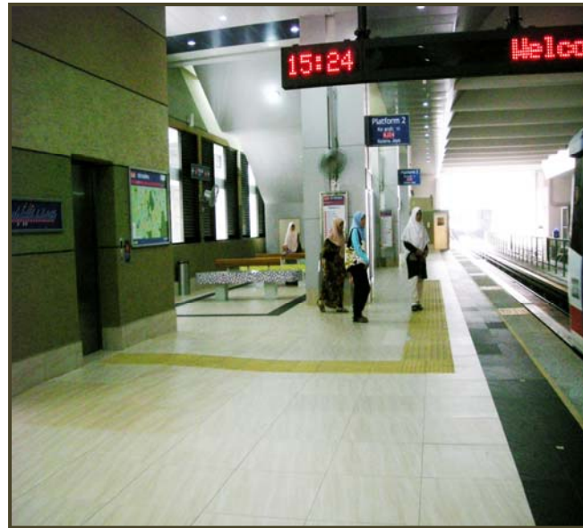
Figure 9: Guiding blocks at the platform area.
