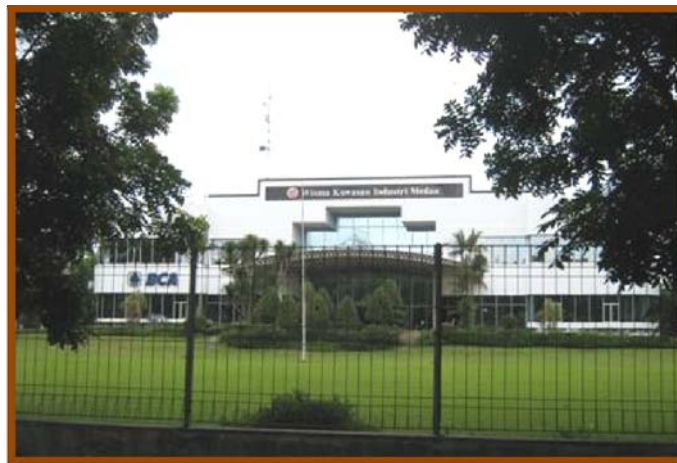
Figure 6: Office Management of Medan Industrial Estate.
