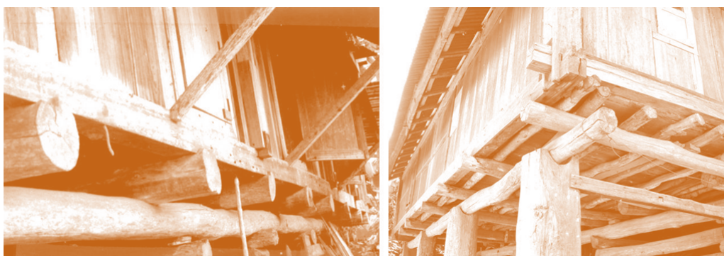
Figure 4: Nail-less timber construction of lamban tuha .
