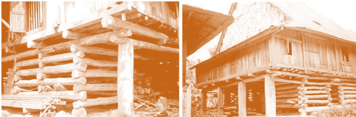
Figure 5: Kalindang of lamban tuha 1 (9 layers) and kalindang lamban tuha 2 (11 layers).
