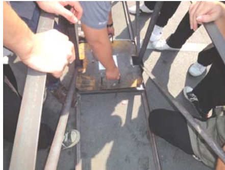
Figure 6: Loading Plate Installation
