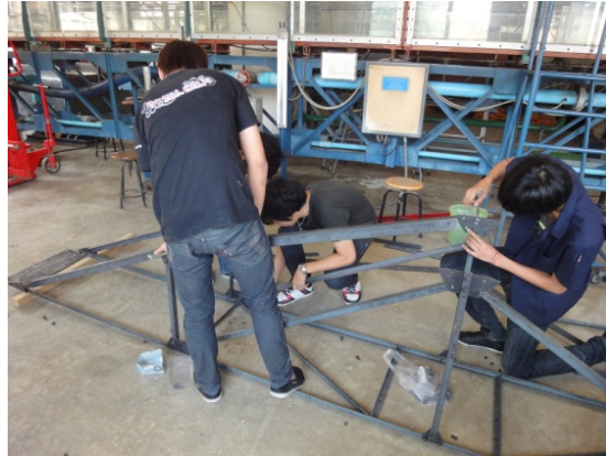
Figure 10: Bridge Structure Joints: TU Bridge Design Team
