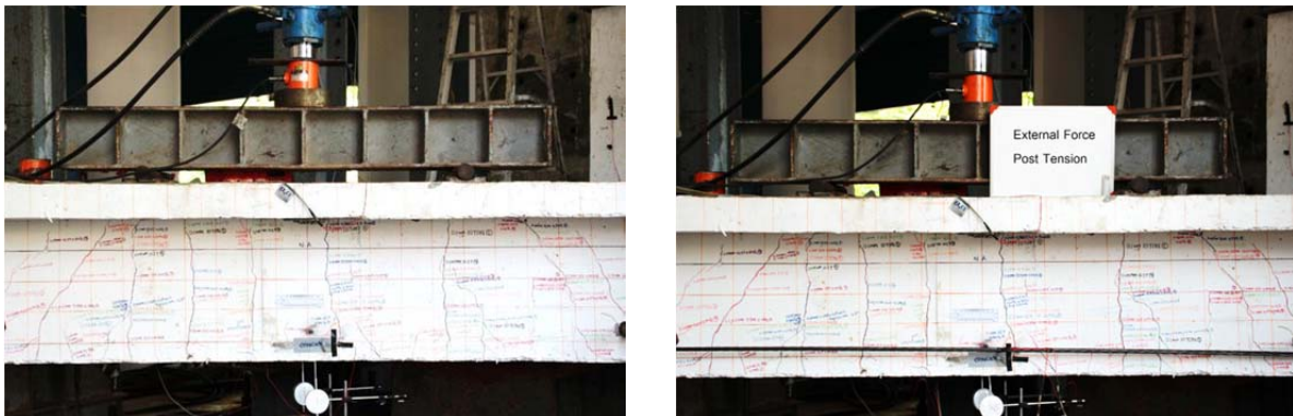
Figure 5: Crack width damage and external post-tension
