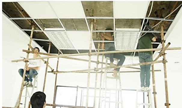
Figure 3: Dial Gauges installation.
