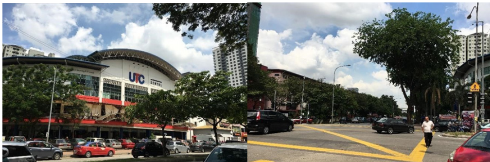
Figure 21: UTC Sentul building (left), site's main intersection (right).
