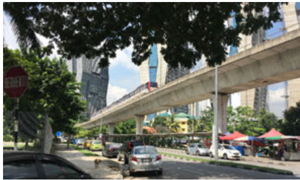
Figure 8: LRT Railway at the west side of Bandar Baru Sentul.
