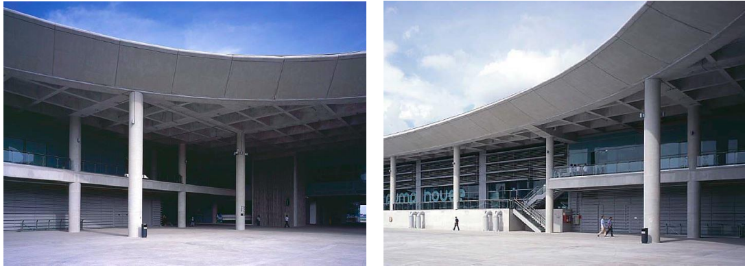
Figure 12: (Left) Sustainable galleries located on the first floor. (Right): Staircase (S1A) connected the ground floor to the first floor. (Source: Darren Soh)
