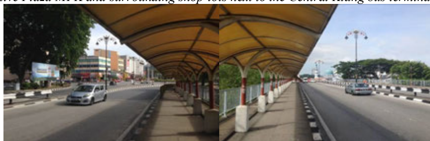
d) Underused pedestrian walkway to KTM (railway) station
