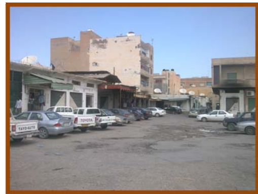
Figure 7: New development is alien to traditional shops in terms of architectural qualities, scale and proportion.
