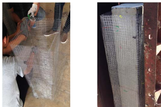
Figure 4: Wrapping of wire mesh before applying mortar cement.
