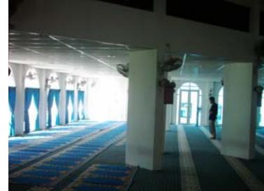
Figure 3: Lower ceiling area with window openings
