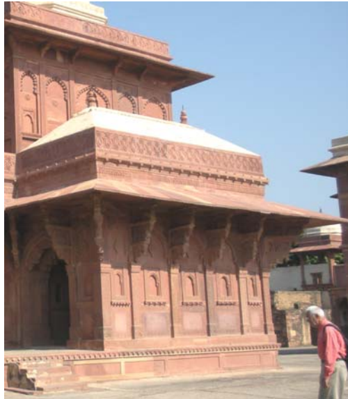
Figure 6: Deep inclined sunshades protect more area of walls and openings from the sun's radiations.
