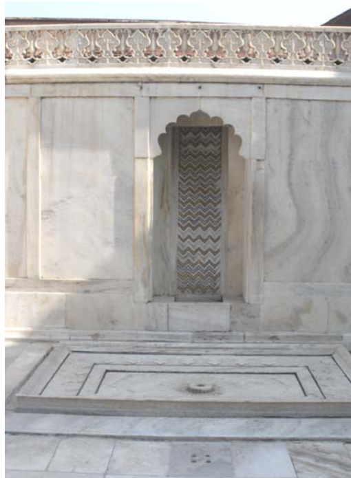
Figure 2: Fountains improve the air quality in a hot dry climate.
