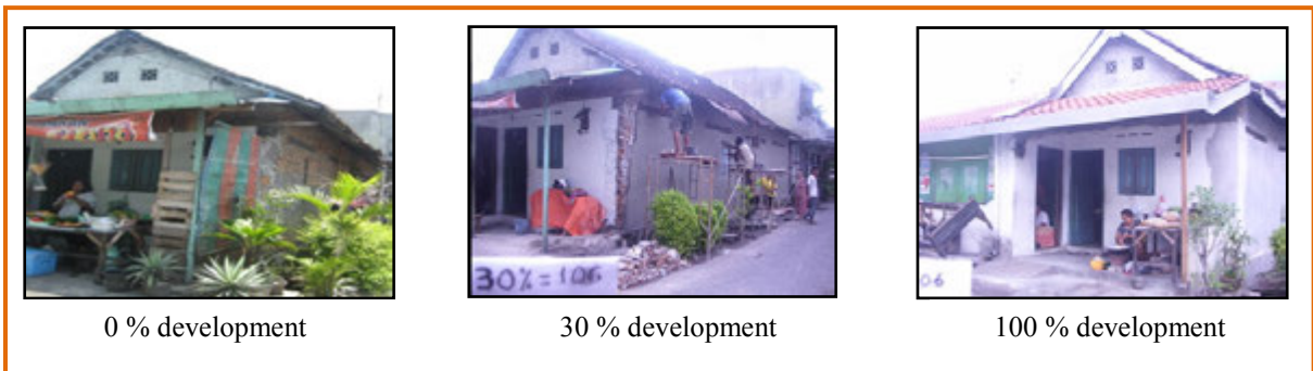
Figure 4: Renovation of Houses (facade, floor and roof).
