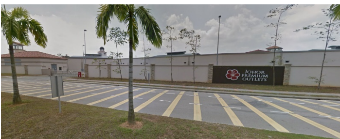
Figure 5: Barrier Wall at Johor Premier Outlet
