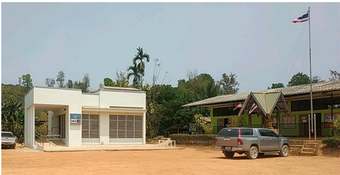
Figure 12: Digital services: Learning centers at schools (Building)
