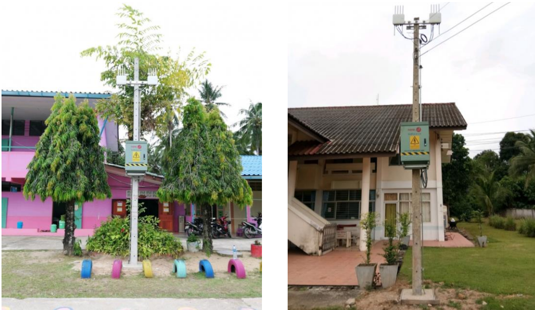
Figure 14: Digital services: Free Wi-Fi services at schools and local hospitals
