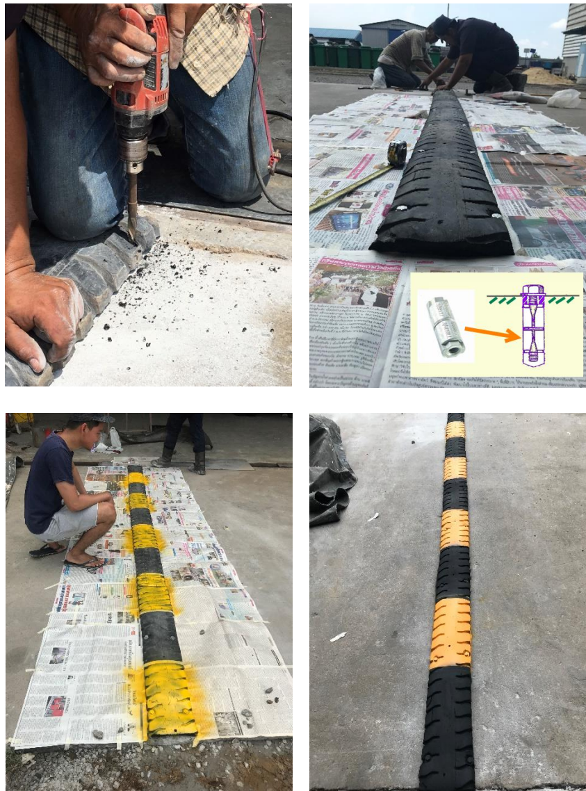
Figure 2: Installation process of bumps built with used pneumatic rubber tires on a local road
