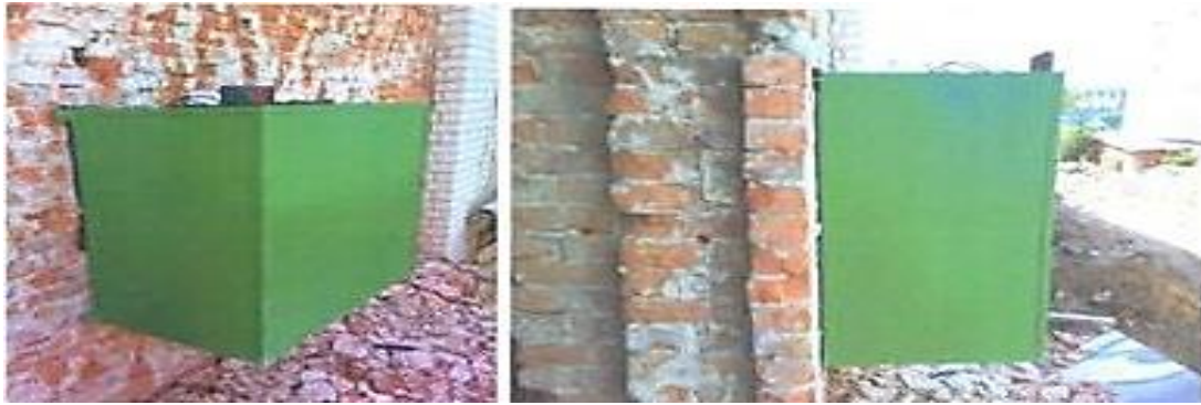
Figure 2: Layout and mounting of the unit to the wall of the object of study
