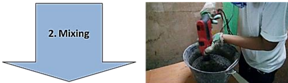
Figure 4: Mixing materials in a bucket.
