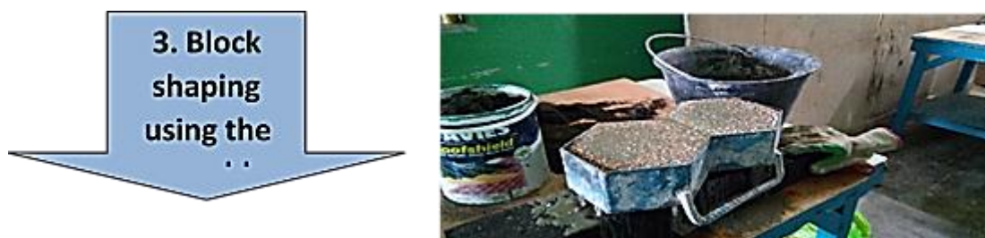
Figure 5: Putting the mixed materials into paver mould.
