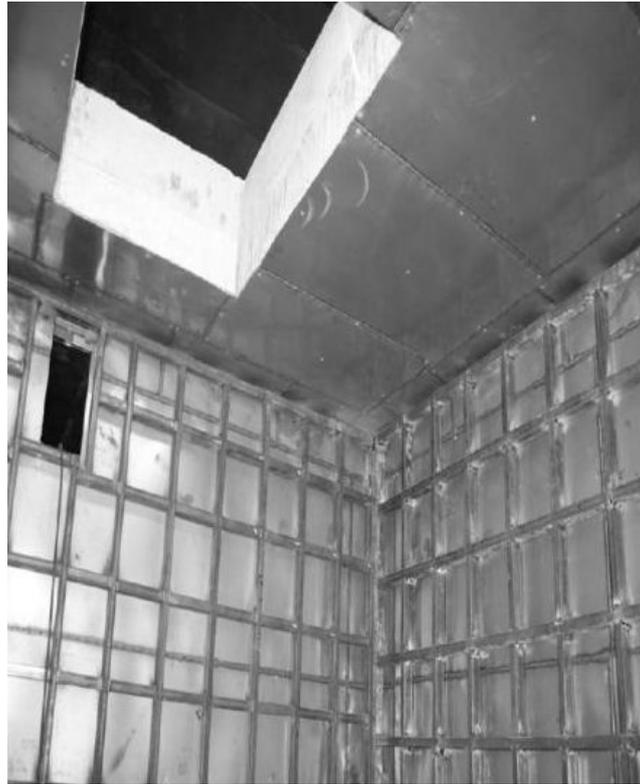
**Figure 5:** Mounting the multilayer shield.
