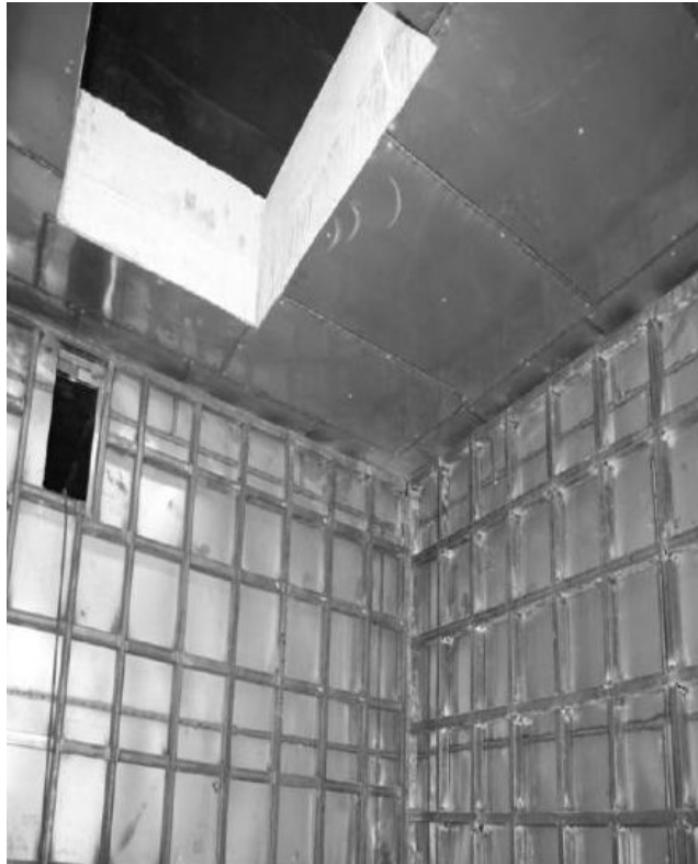
Figure 5: Mounting the multilayer shield.
