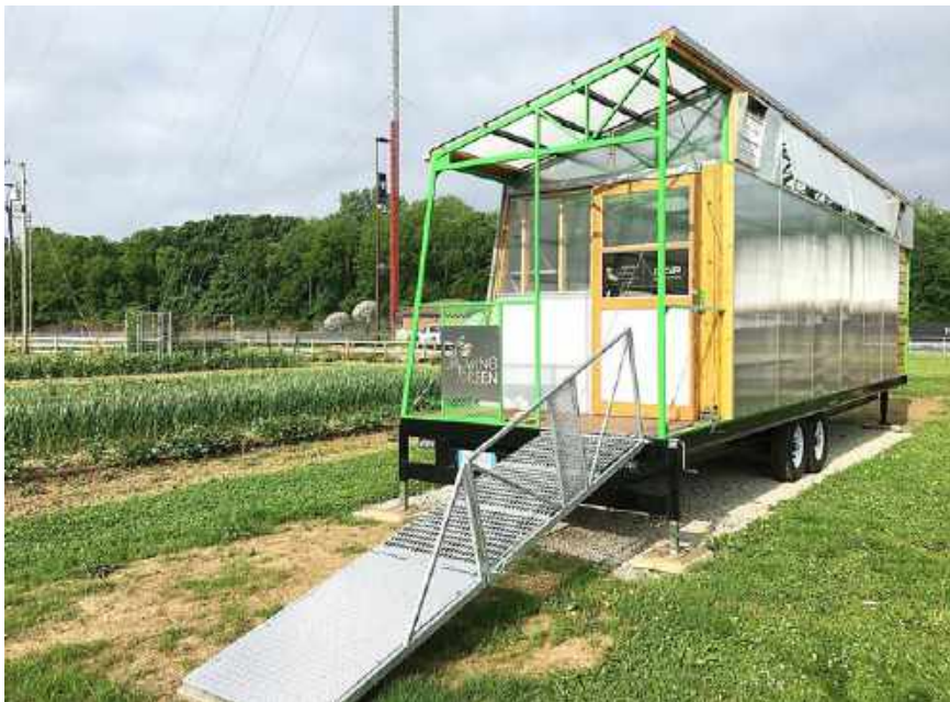
Figure 1: The mobile greenhouse on-site at the Center for Urban Ecology farm shortly after being transported over sixty miles by a standard pickup truck. Sited in the floodplain mobility allows the structure to be legally installed.
