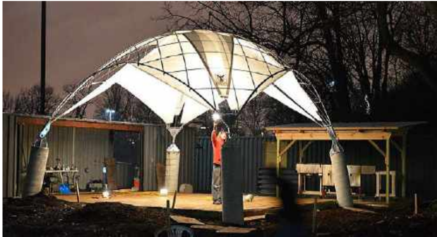
Figure 2: Construction nearing completion on the Gridshell dome at the GRIDfarm, spanning close to 30 feet using only one-inch rebar and clad with a double layer of fabric “sails” made from salvaged material.
