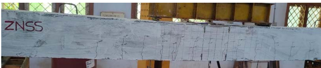
(c) Crack Pattern of ZNSS.
