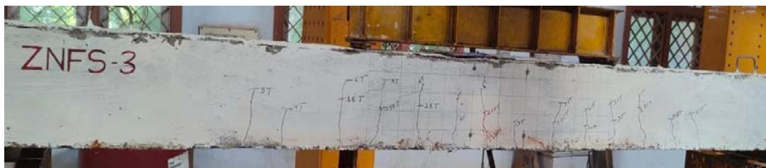
(f) Crack Pattern of ZNFS-3
