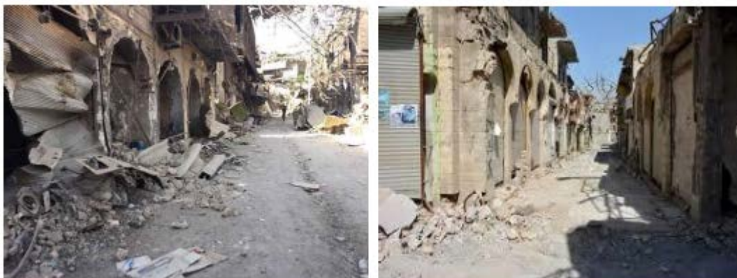
Figure 1: Images of Al-Najafi Street after the war before the reconstruction process in 2017
