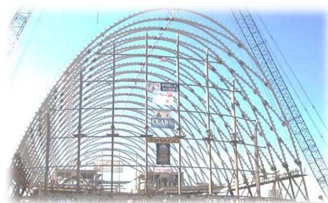
(c) The main sheltered entrance of Anaheim transportation from the construction
