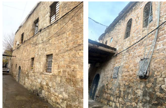
Figure 9: Location of the Doors in Traditional Dwellings.
